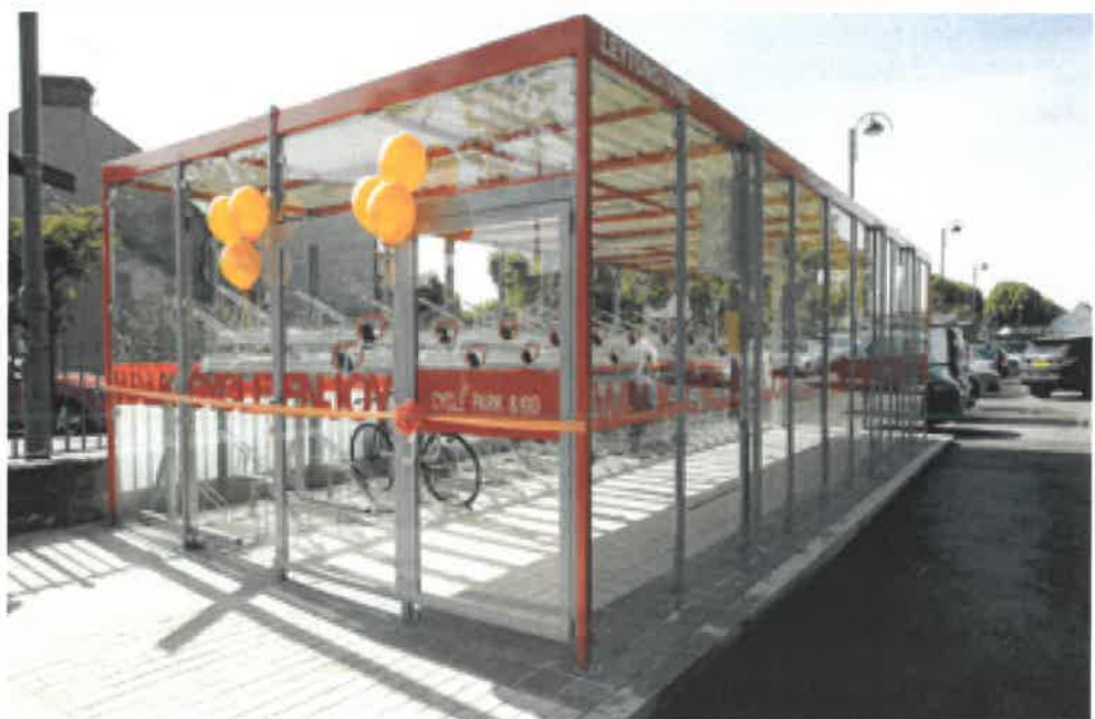
Example of covered secure cycle parking installed in the London Borough of Waltham Forest
