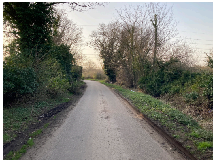
10. Potential for an additional link route above existing drainage ditch (ditch to be culverted) to connect to existing recreational route
