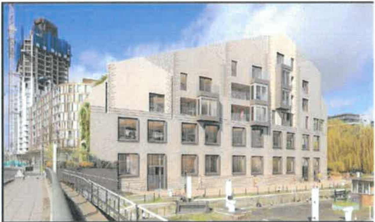
View from Ferry Lane looking at eastern elevation and towpath
