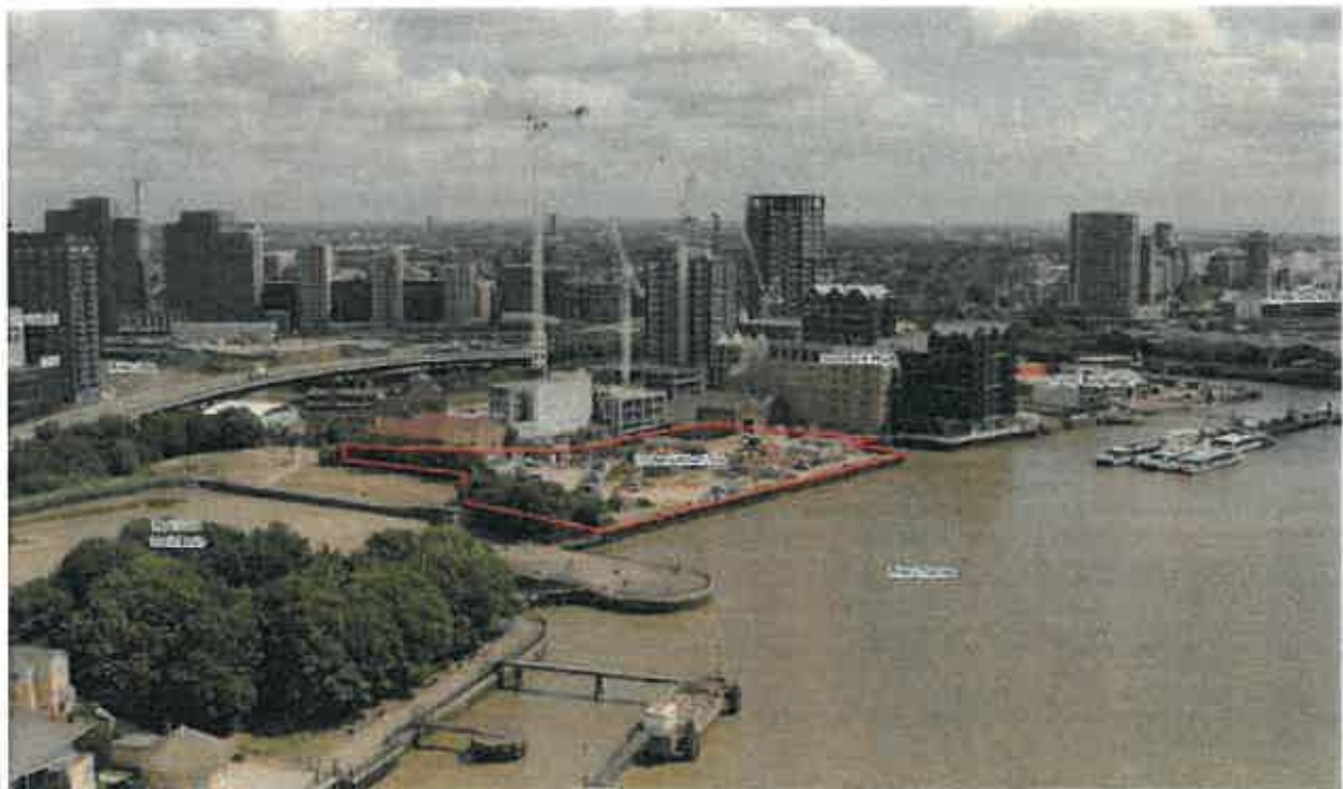
Looking east with EIDB in foreground front left.
