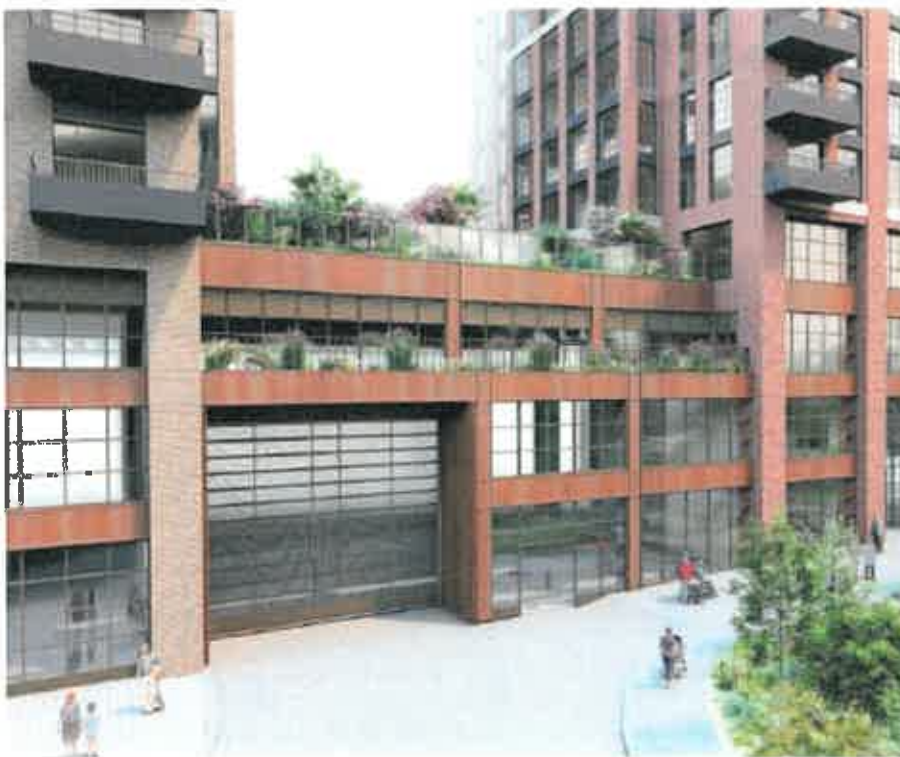
Entrance to Block B from Orchard Place
