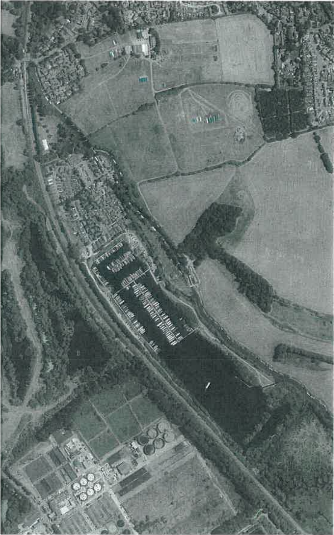
Appendix B Plan Extract from Landscape and Visual Assessment showing existing marina
