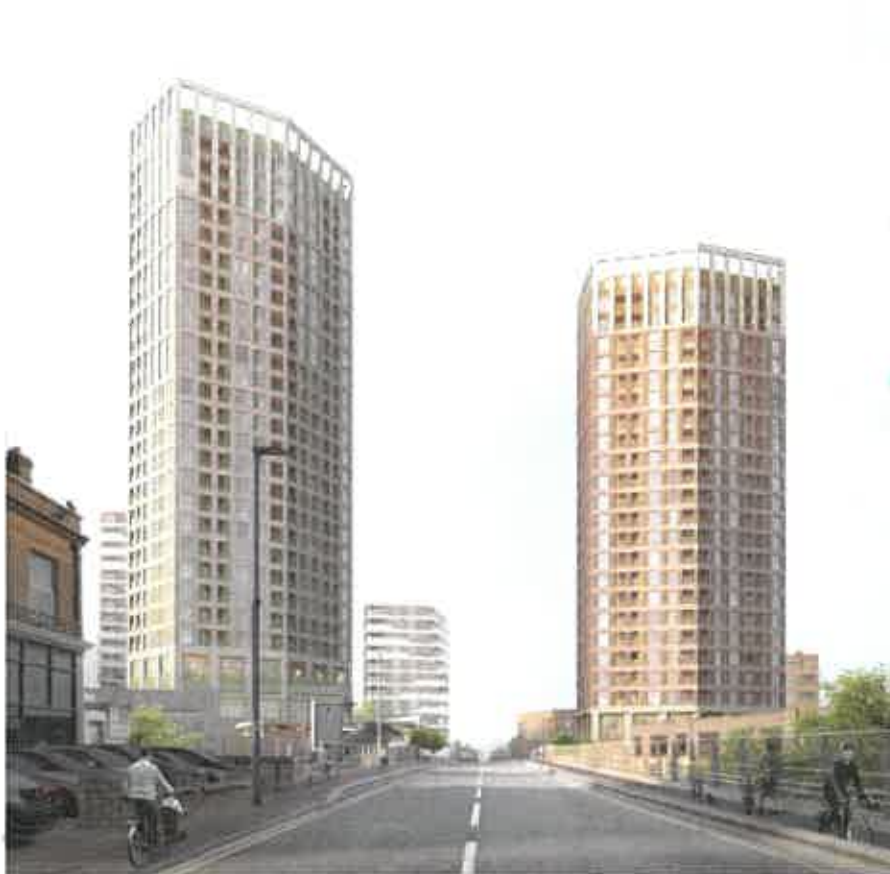
Above - View of Tower 1 and 2 from Lea Bridge Road looking east.
