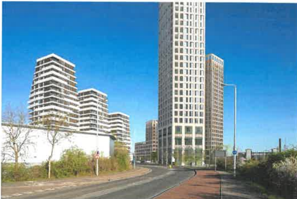
View 15 south from Argall Way – Lea Bridge Station on the right
